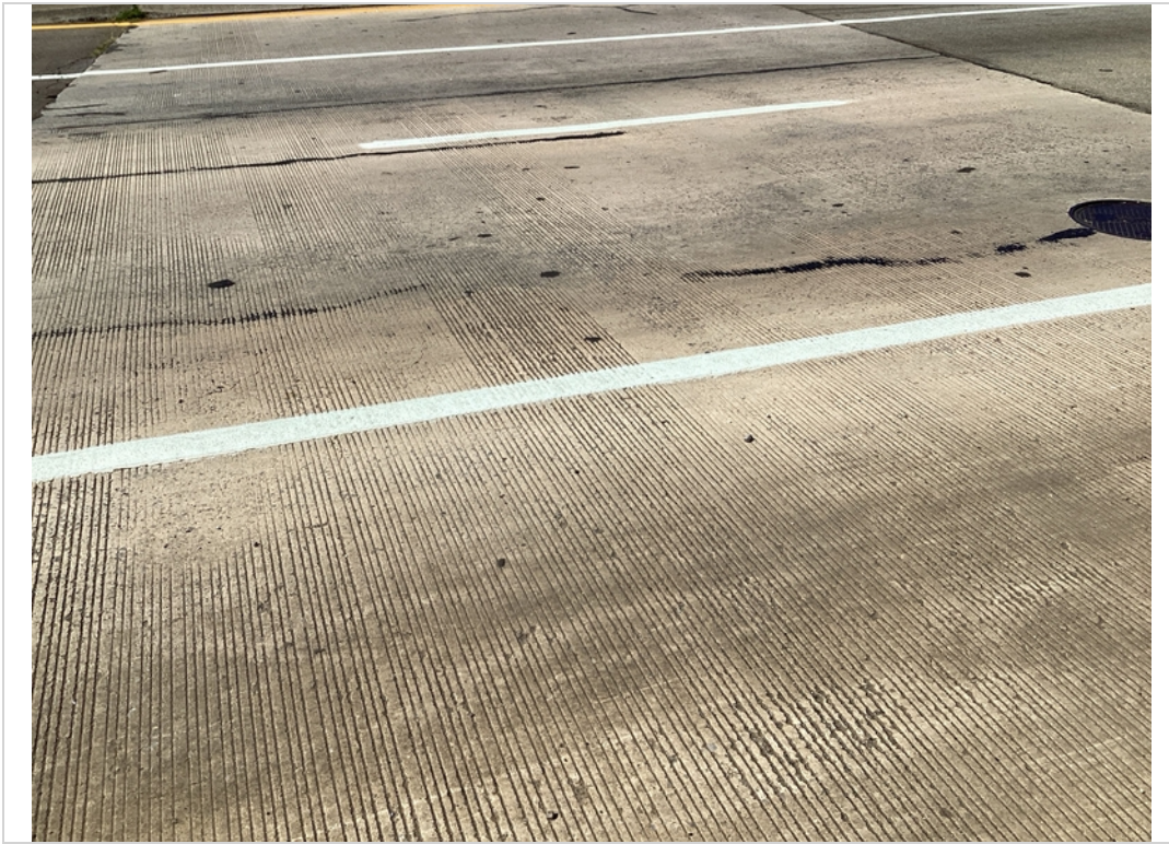
Approach 2 slab left lane - hairline cracks sealed
