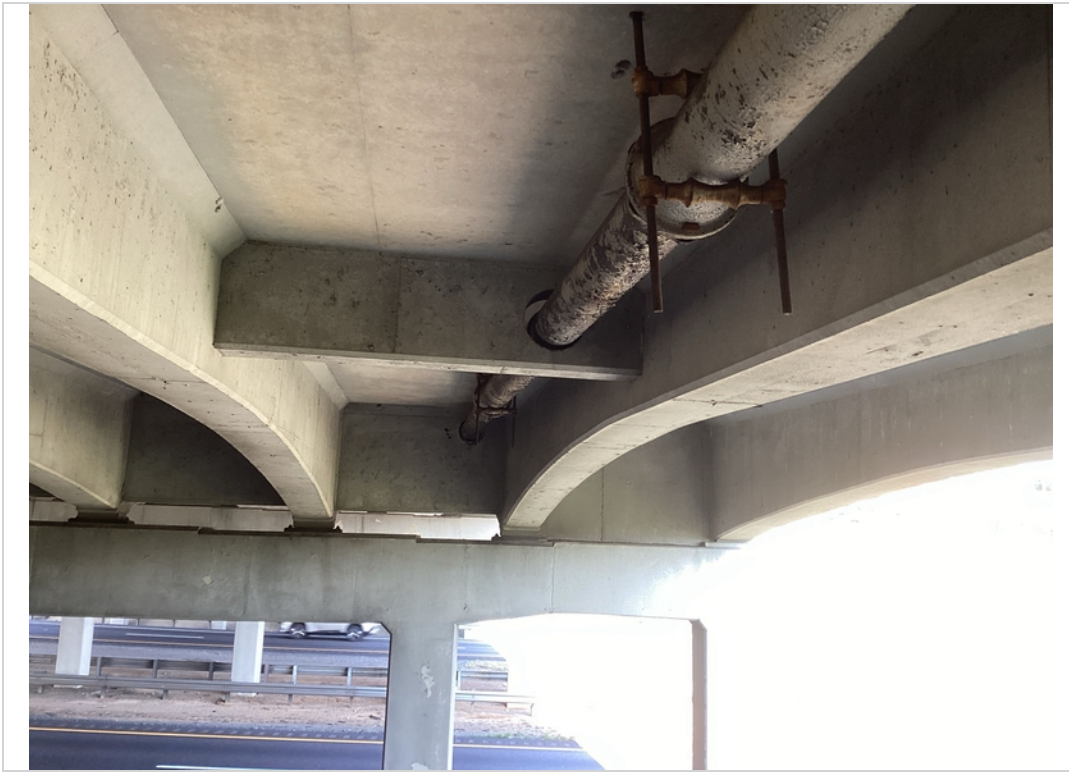
Between beams B/C - Utility
