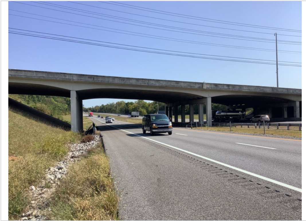
I-75 SB - Underpass forward
