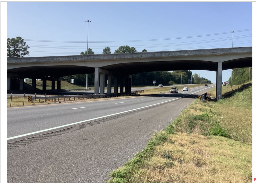
I-75 SB - Underpass back
