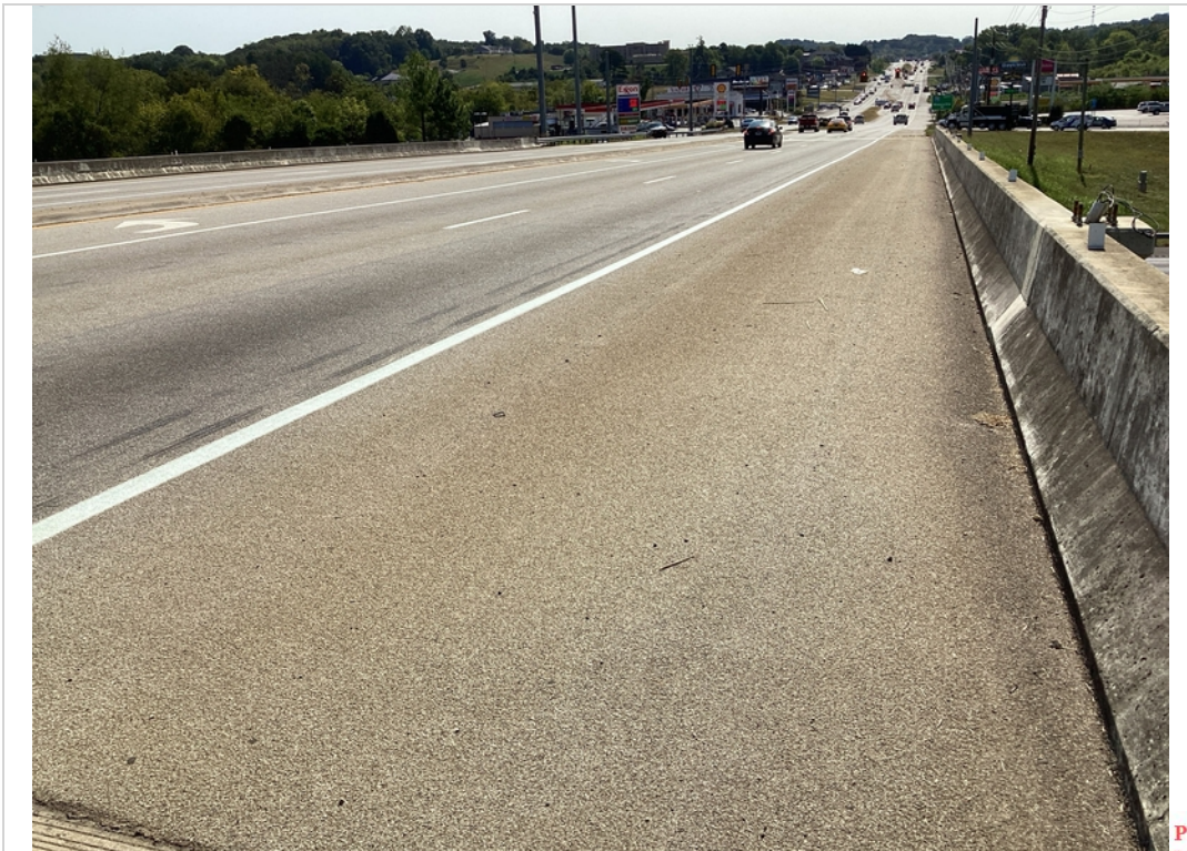
View across deck right lane
