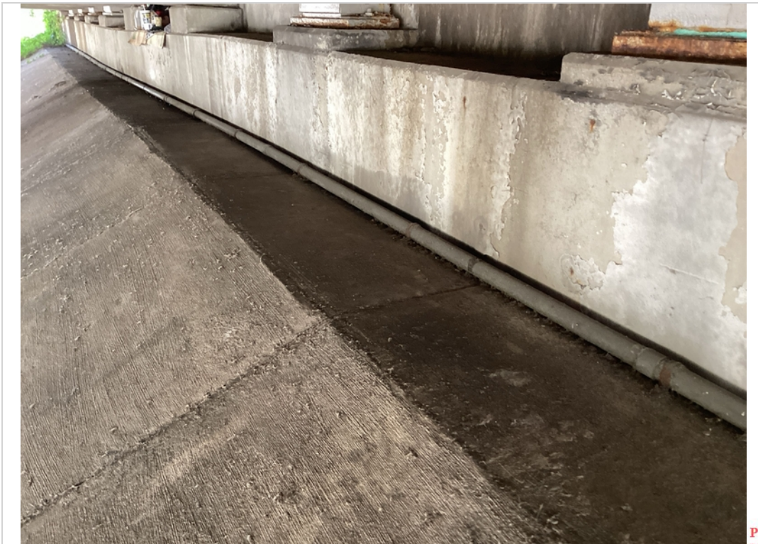
Abutment 2 - utilities on both abutments
