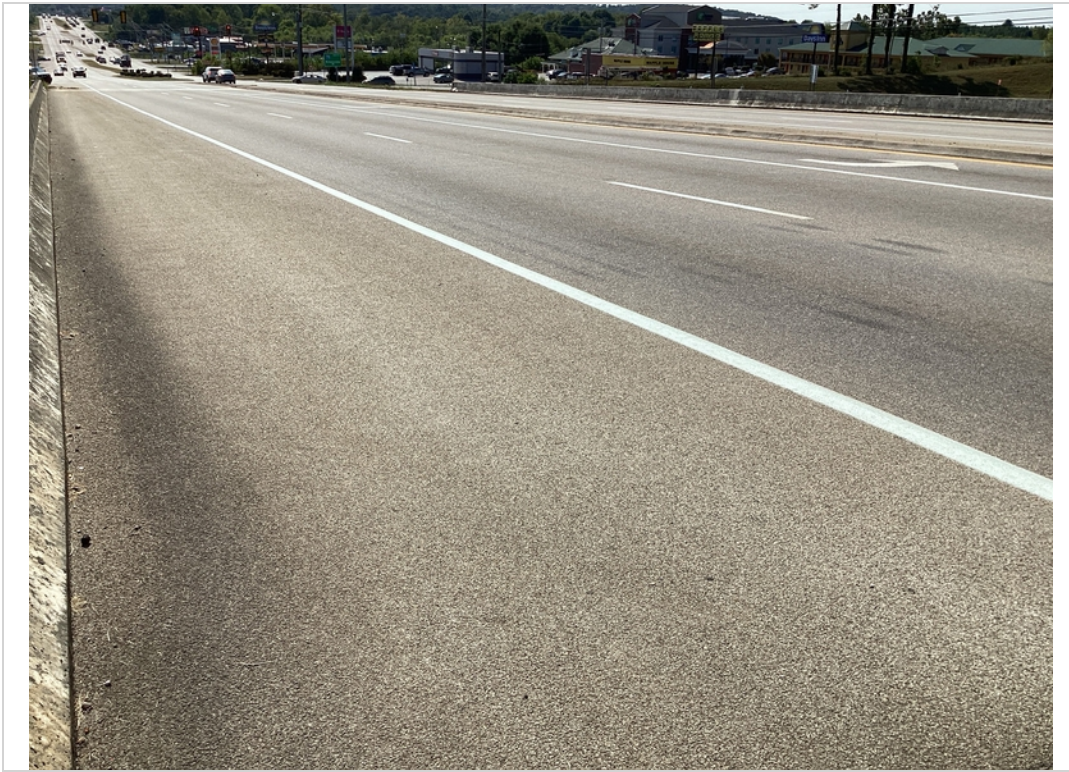
View across deck left lane
