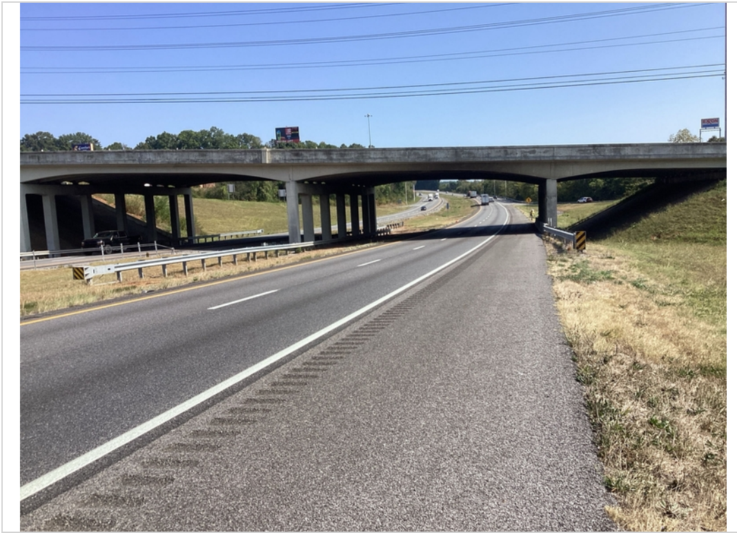
I-75 NB - Underpass - Approach forward on log
